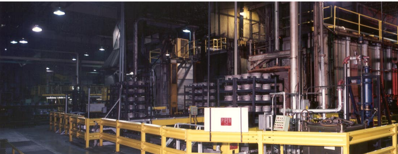
Roller Hearth Solution Heat Treat Line
